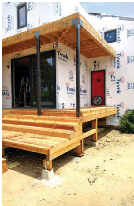
Perlita Passive House in Los Angeles, CA designed by Arcolution LLC. A blower door test is conducted to quantify the amount of air leakage and the effectiveness the air-sealing prior to finishing the house. (Image courtesy of Lawrence Anderson)
