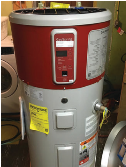
Individual heat pump water heater. The heat pump is located above the storage tank (Courtesy Jeff Robbins).
