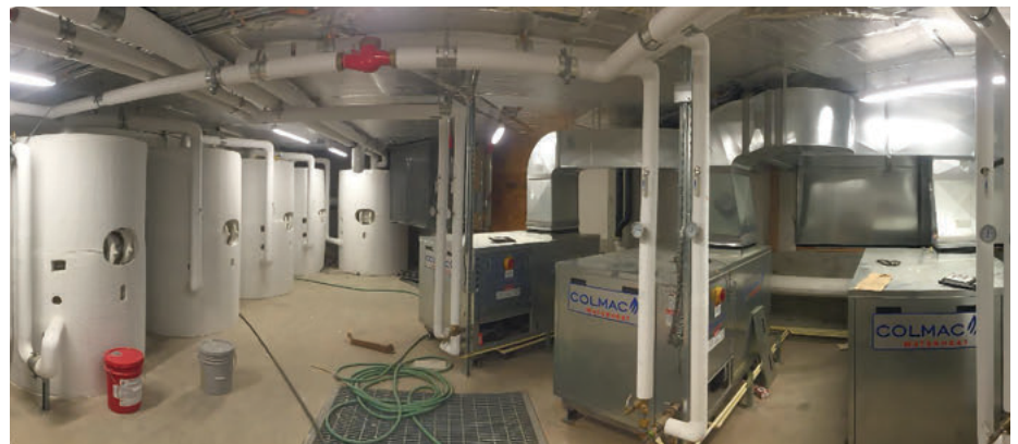
Central HPWH equipment with 2500 gallons storage located in a parking garage in the Batik Apartments, Seattle, WA (Courtesy of Ecotope).
