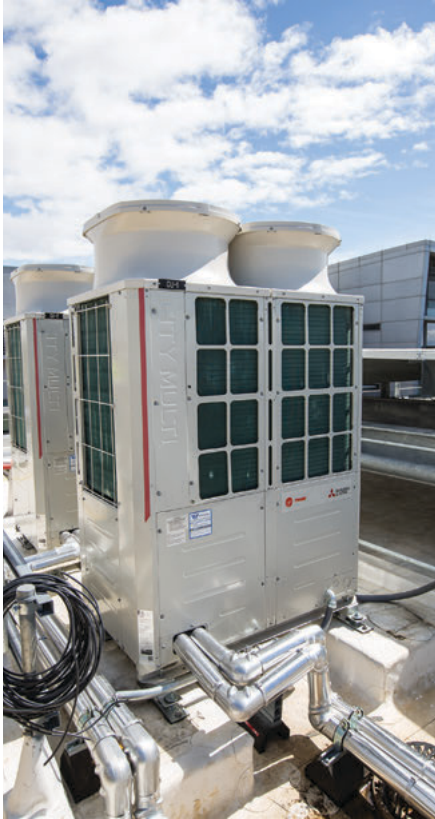
The outdoor unit for a commercial heat pump space conditioning system at the Santa Monica City Hall (Courtesy of City of Santa Monica).
