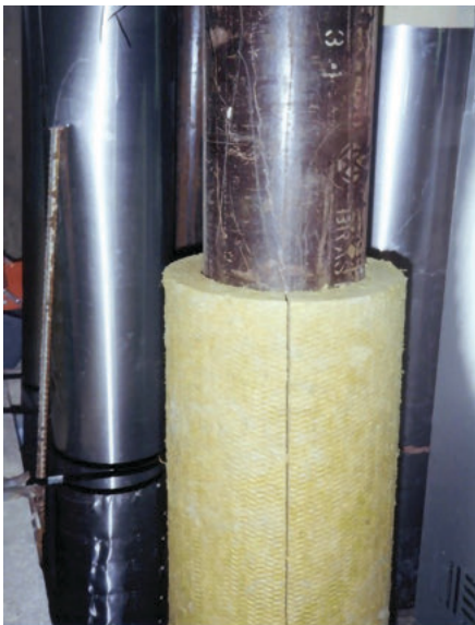
Insulating pipes reduces heat loss in pipes (Courtesy Wikipedia).
