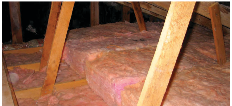
R-38 Attic Insulation. Photo by Ryan McFarland. www.zieak.com
