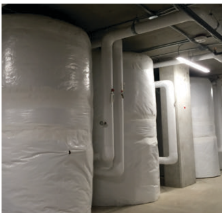
2500 Gallons of Well-Insulated Storage for Cyprus Apartments – 230 Market Rate Units (Courtesy of Ecotope).
